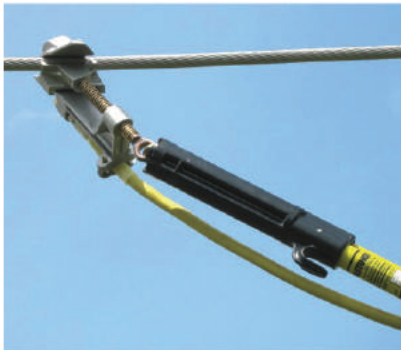
INSTALLING CLAMP
